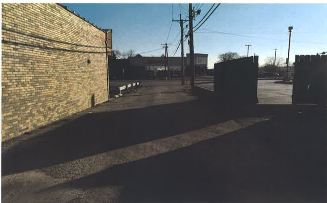
VIEW EAST ALONG THE SUBJECT ALLEY
