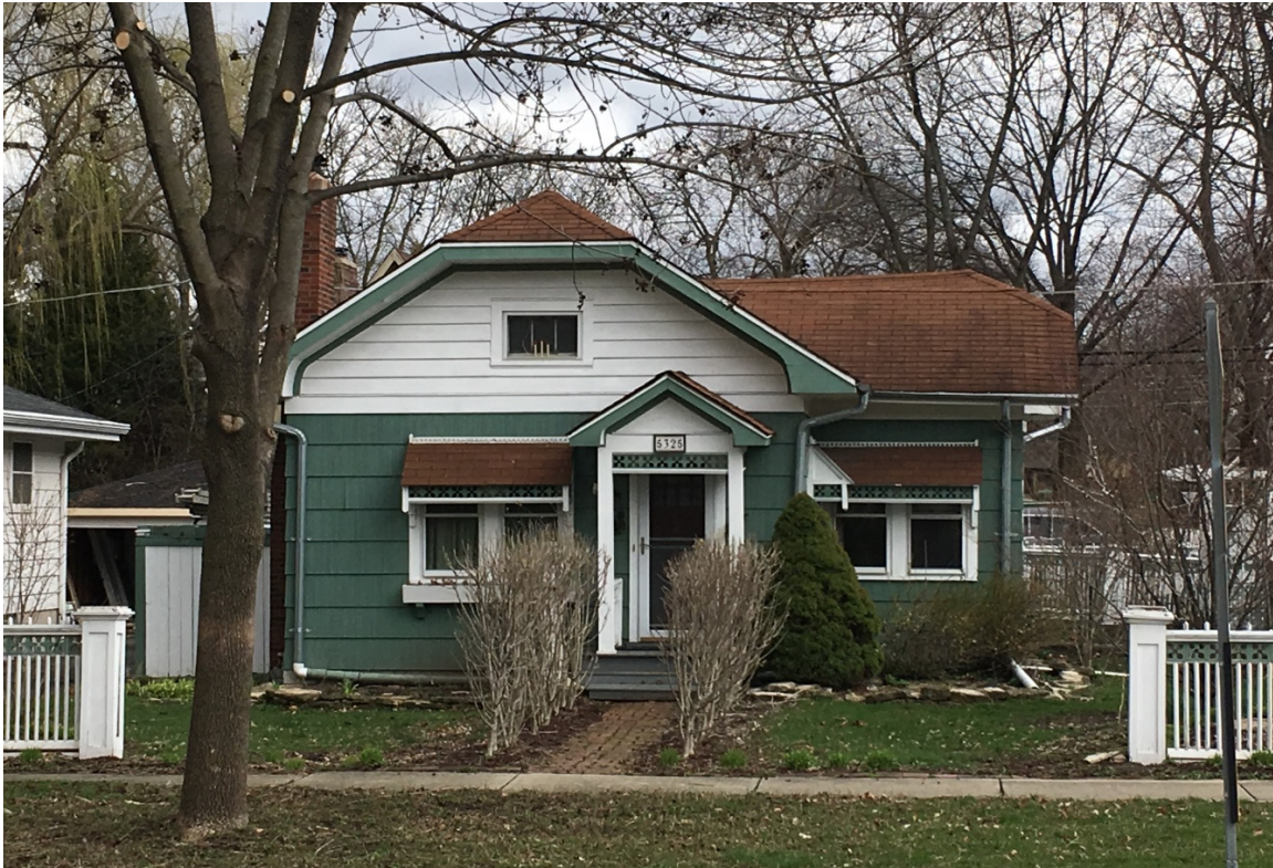
Photo #1: Front (East) Elevation – April 4, 2017
