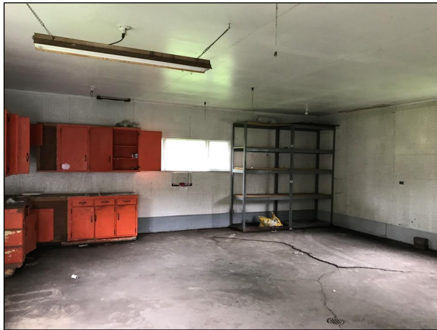
Photograph 6 – A view of the interior of the garage.
