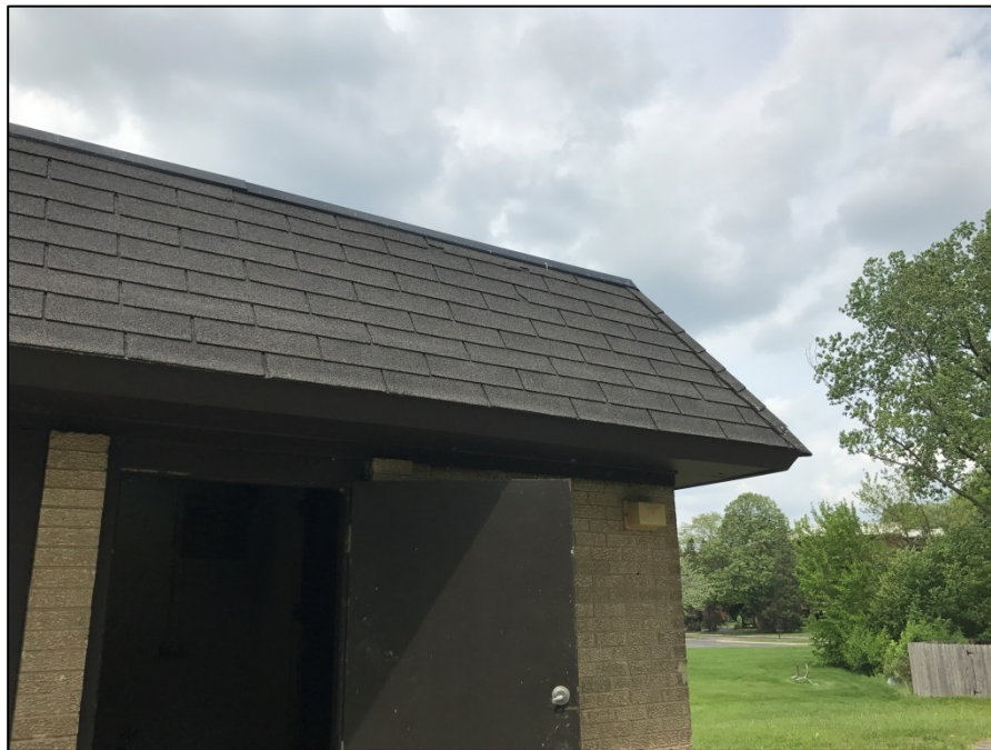
Photograph 4 – A view of the rooftop showing the asbestos containing shingles.
