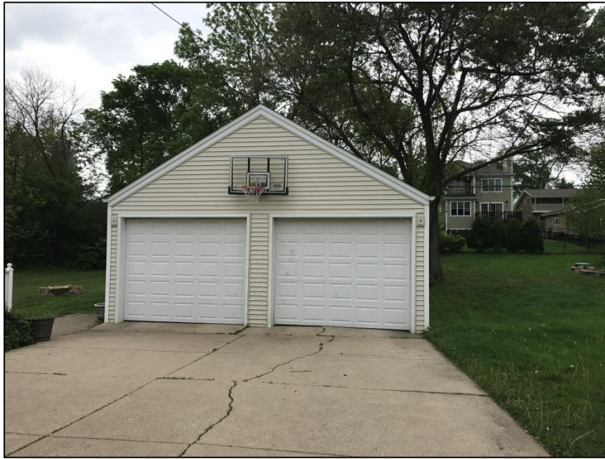
Photograph 5 – A view of the exterior of the garage.
