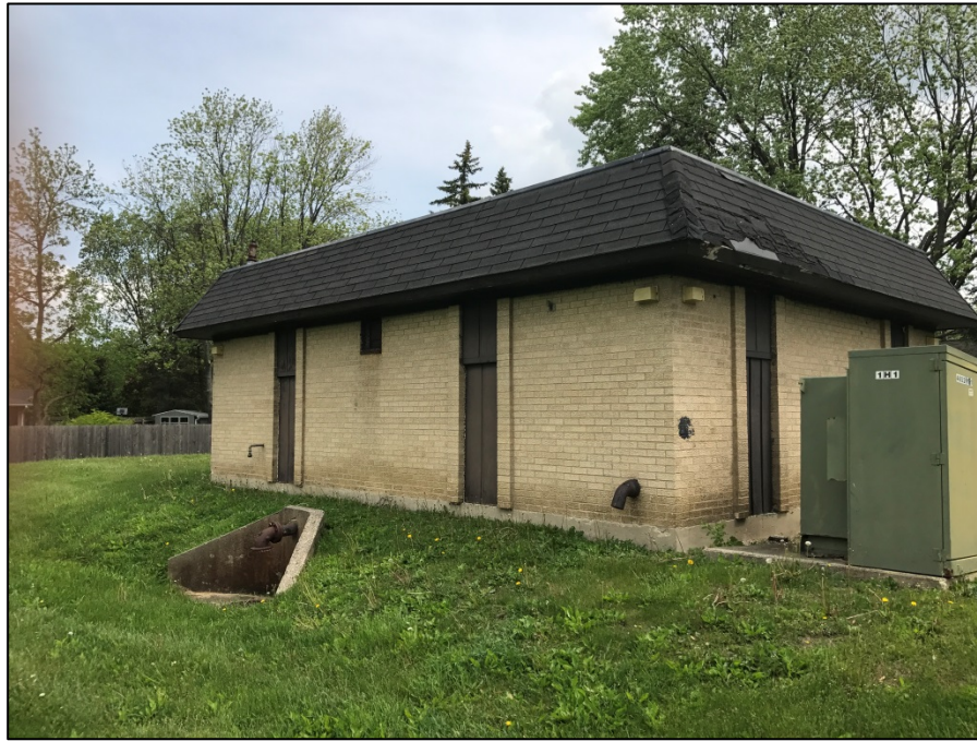
Photograph 1 – A view of the building at 926 67 th Street.
