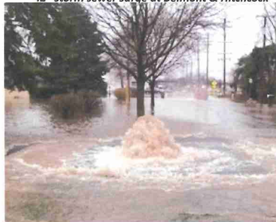
42" storm sewer surge at Belmont & Hitchcock
