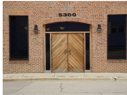
Fig. 10: Opaque windows and windows which do not make up the majority of the storefront are discouraged and should be avoided.
