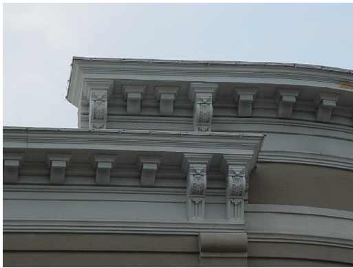
Fig. 37: Encouraged: cornice detailing
