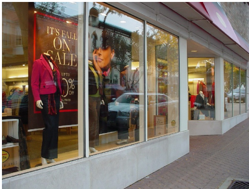
Fig. 7: Encouraged: knee walls and windows which make up a majority of the storefront
