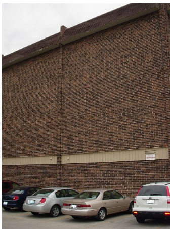
Fig. 32: Blank façades with no variation, windows or detailing should be avoided
