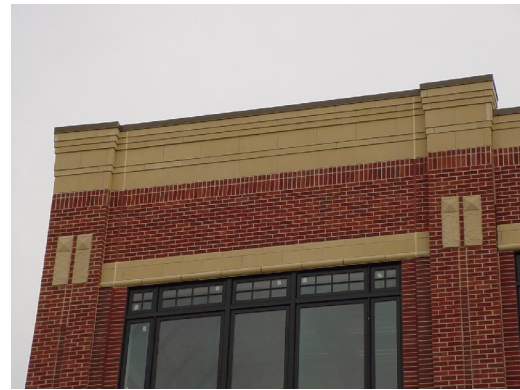
Fig. 38: Encouraged: stone cornice detailing
