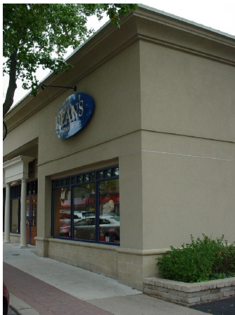
Fig. 17: Materials such as EIFS can be used effectively as an accent. However, it is discouraged as a primary material
