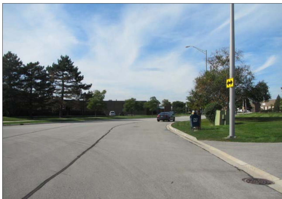
BROOK DRIVE LOOKING WEST AT DOWNERS DRIVE
