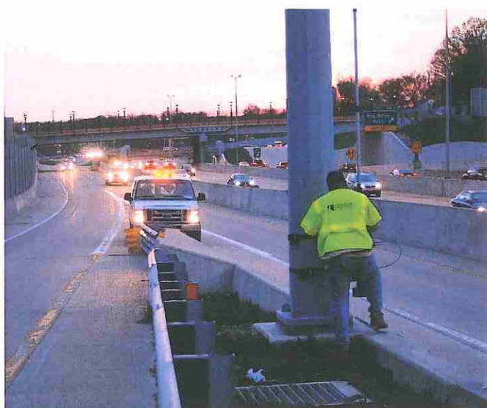
A TERRA team member installs a Miovision camera for traffic data collection
