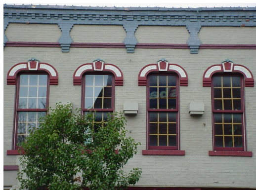
Fig. 27: Encouraged: replacement windows that fill the entire window opening
