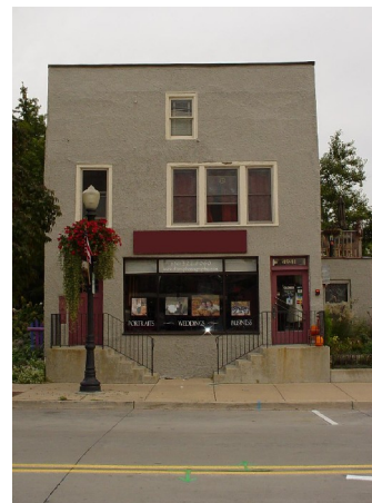
Fig. 33: Façades with no detailing, as in this example, should be avoided
