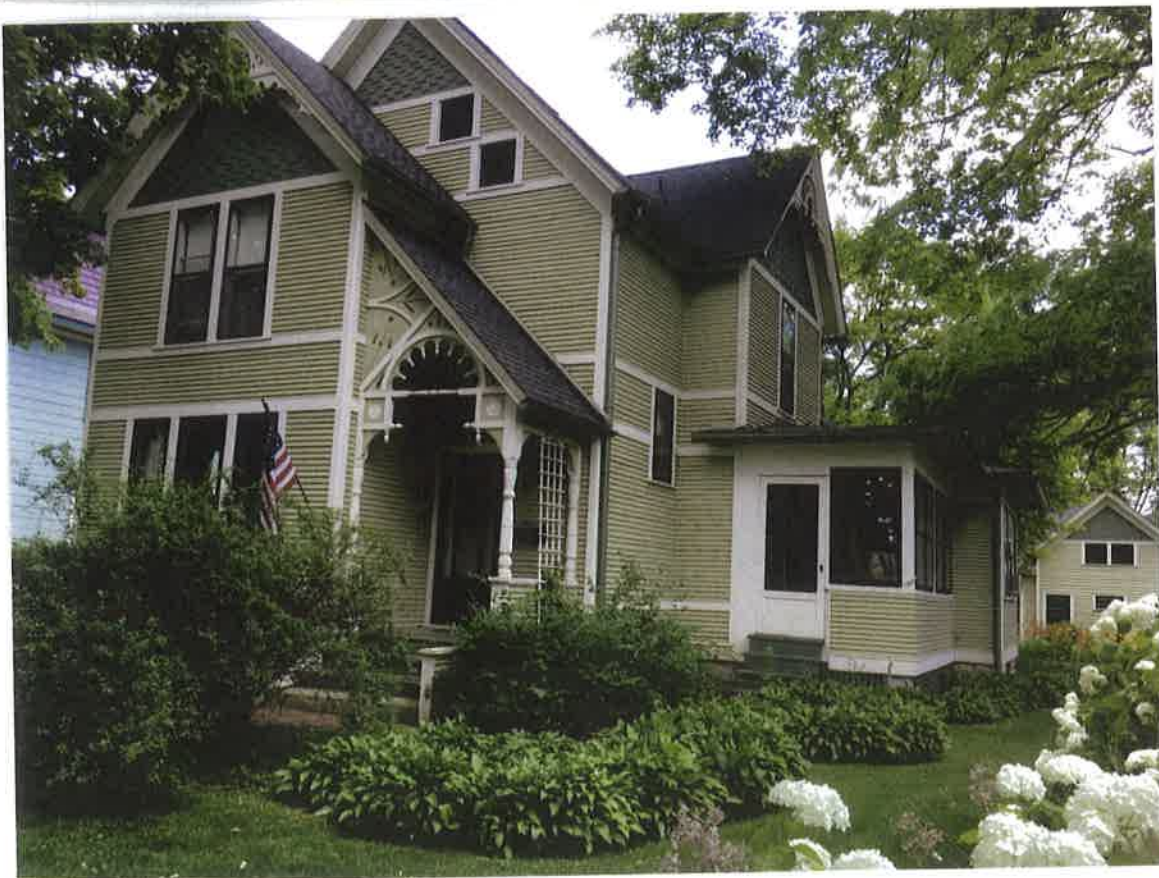
side front view
