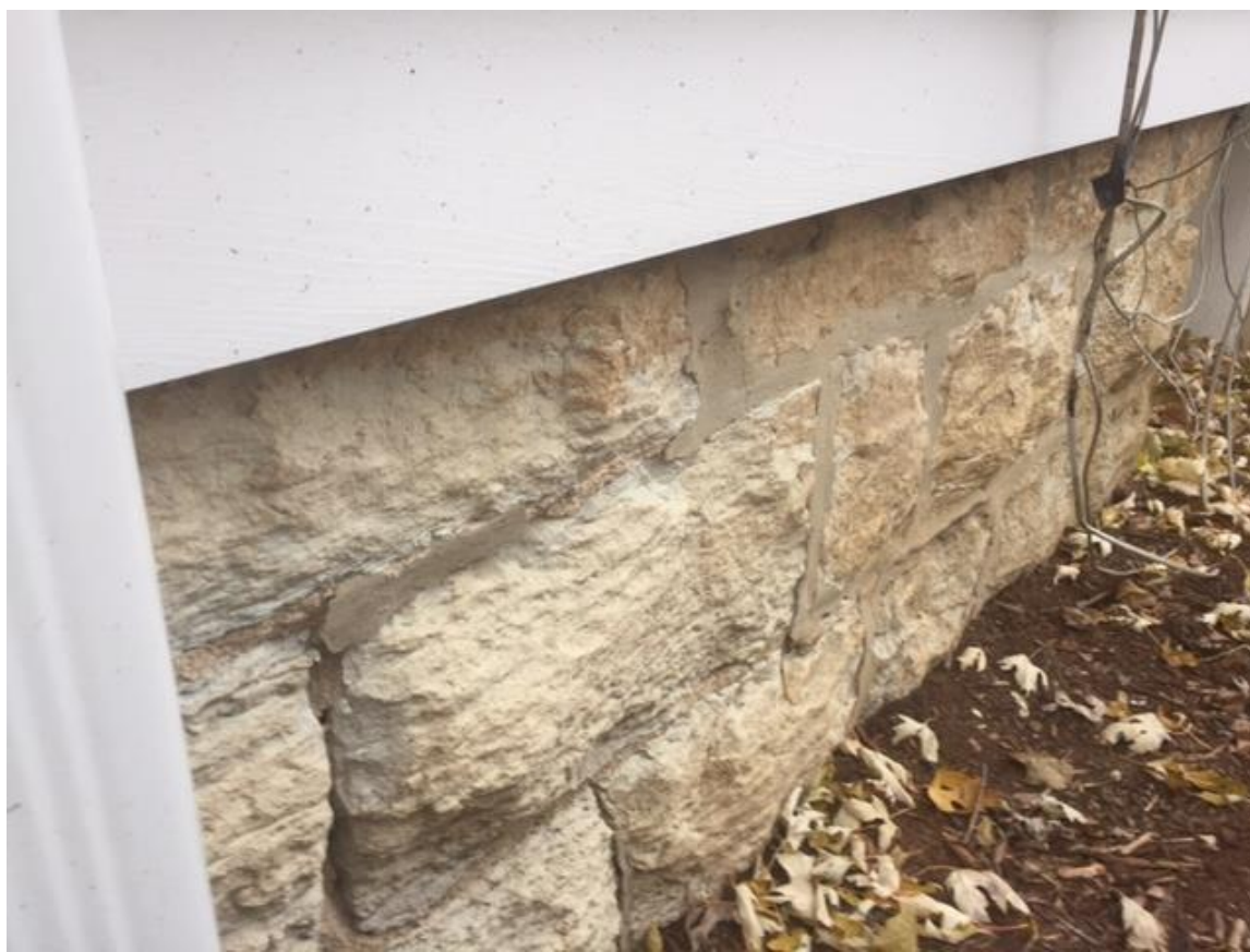
Original stone foundation.
