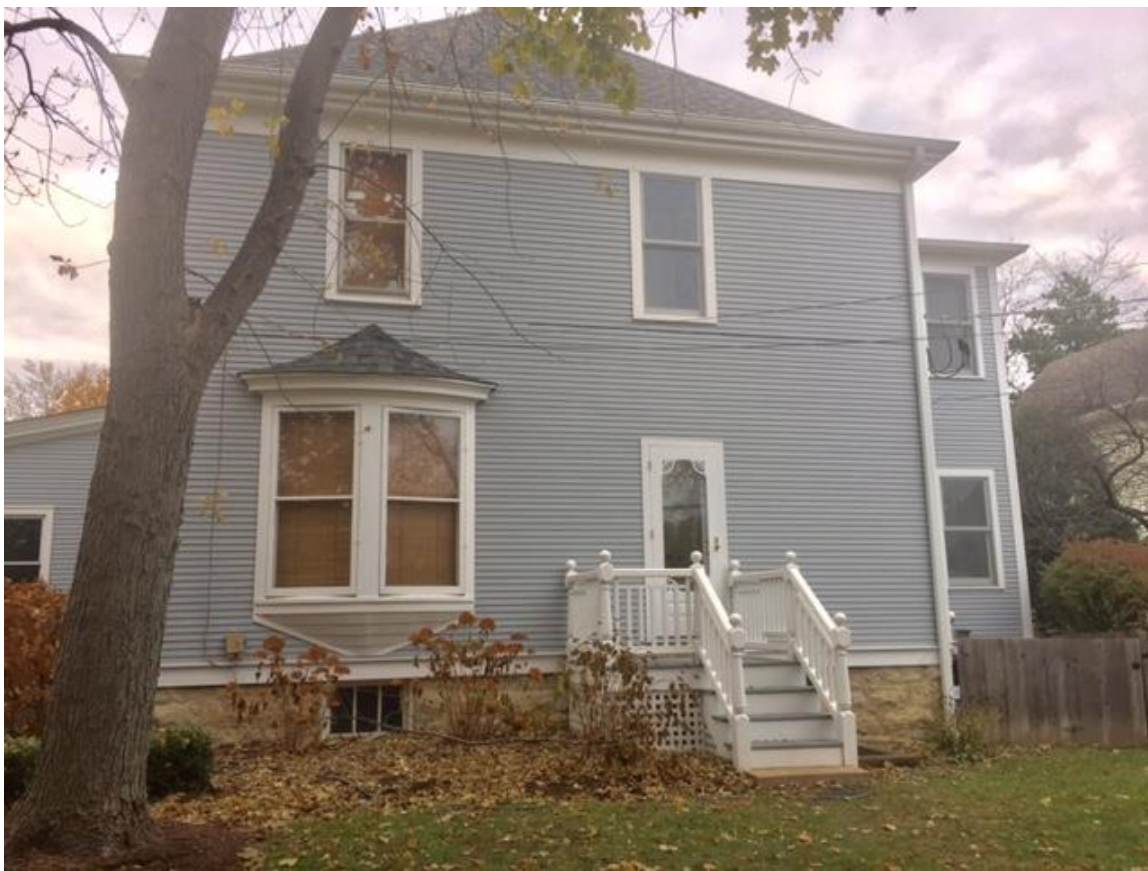
West view – Outstanding oriel window. Decorative porch with lattice and hipped roofline.
