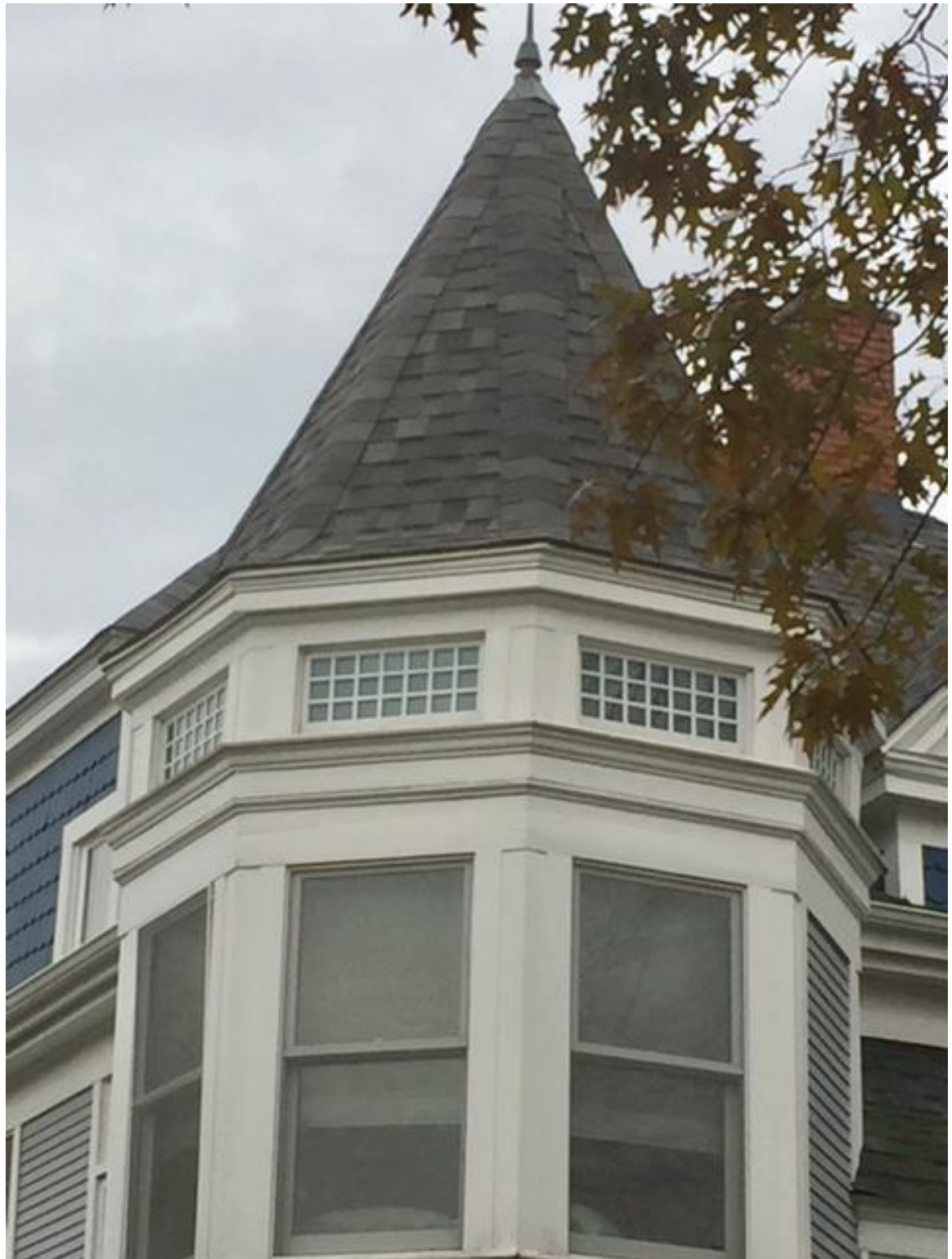
Turret windows and decorative soffits.
