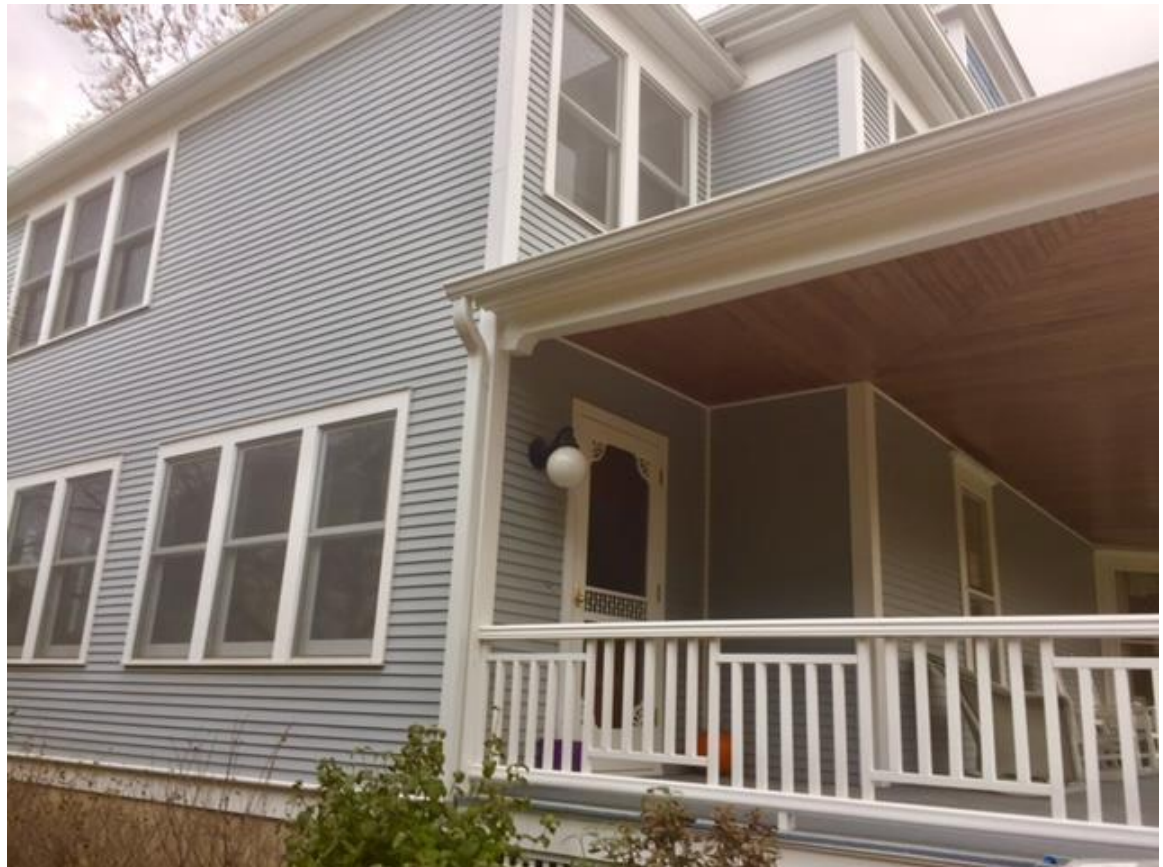
South view addition. Nice view of porch work.
