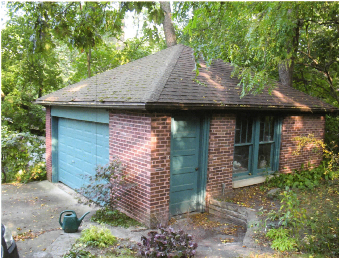
Photo #10: Garage – view from Northwest – 9/12/2017
