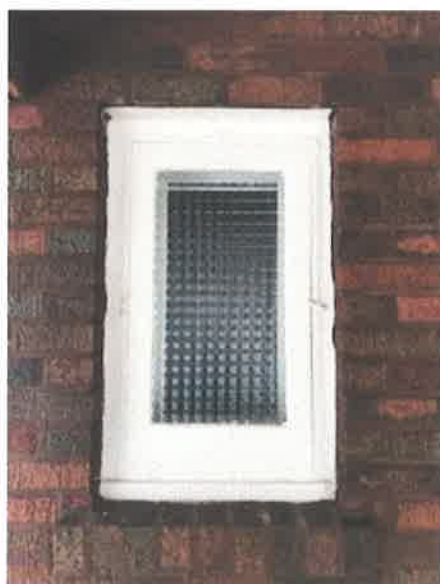
Original porch window
