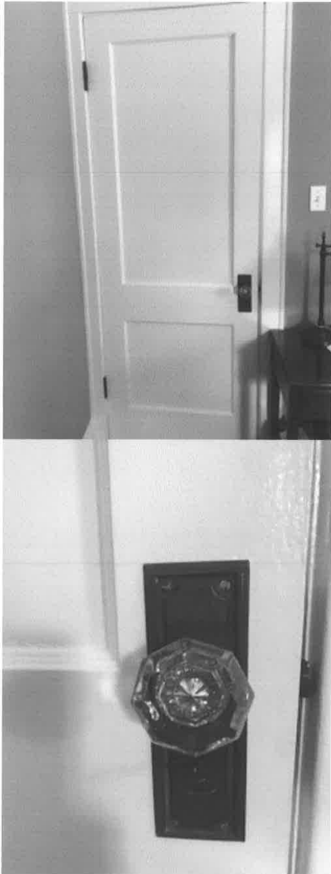
Example of an Interior Door- original with Original hardware
