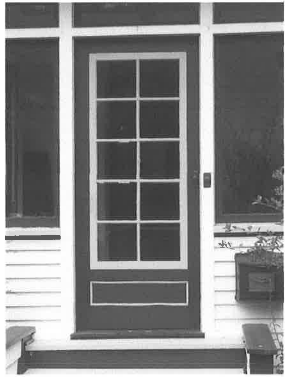
Photo #5: Original storm door at front entry
