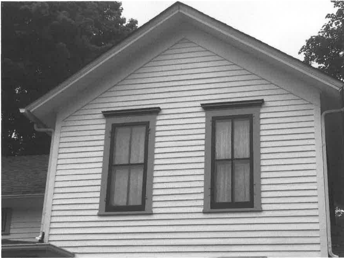
Photo #3: Original wood clapboard siding and wide trim under gable
