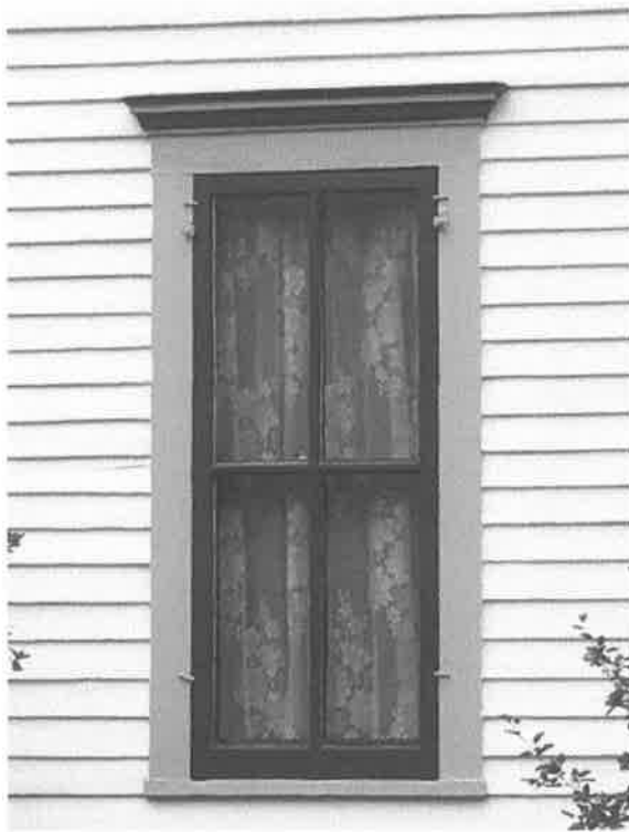
Photo #4: Original double hung window, storm window, wood trim and window hood molding
