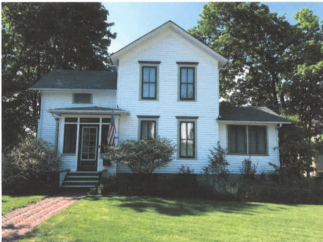
Photo #1: Front (South) Elevation – 5/27/2018
