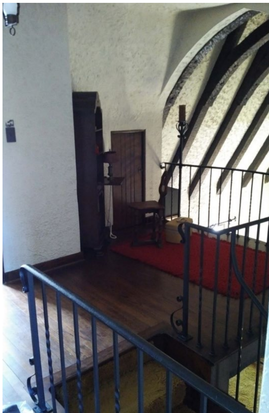
Figure 10 – Representative Wrought Iron Railings on Balcony
