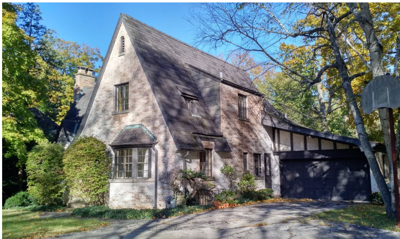
Figure 2 – Elevation View Looking to the Northwest
