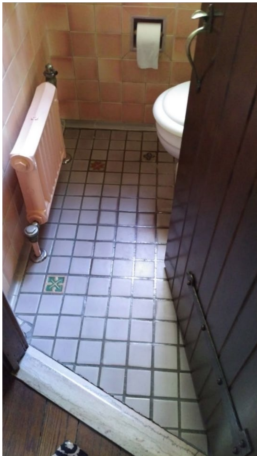
Figure 11 – Room and Floor Tile
