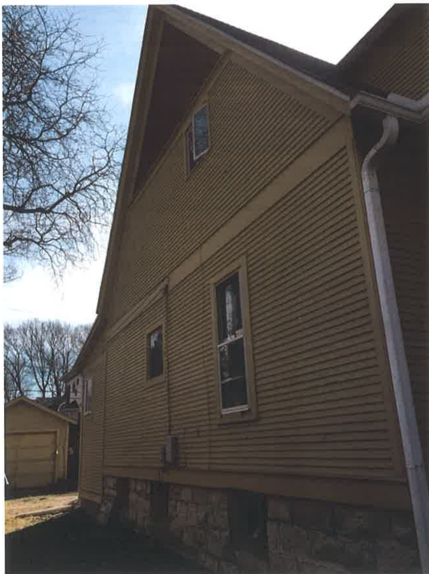
Photo #2: Side elevation facing north, April 2, 2019.
