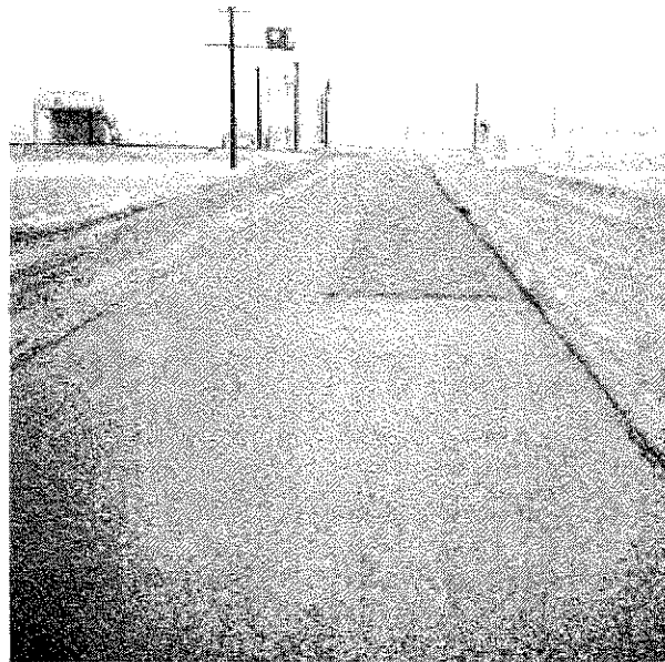
April, 1971—21 Months after Reclamite Treatment. (2 Hours after Rain)
