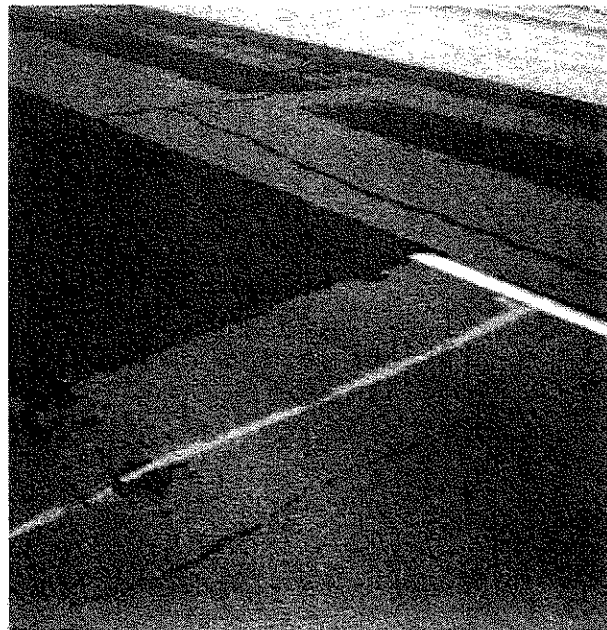
8. Close-up of drying pavement at beginning of test section.
