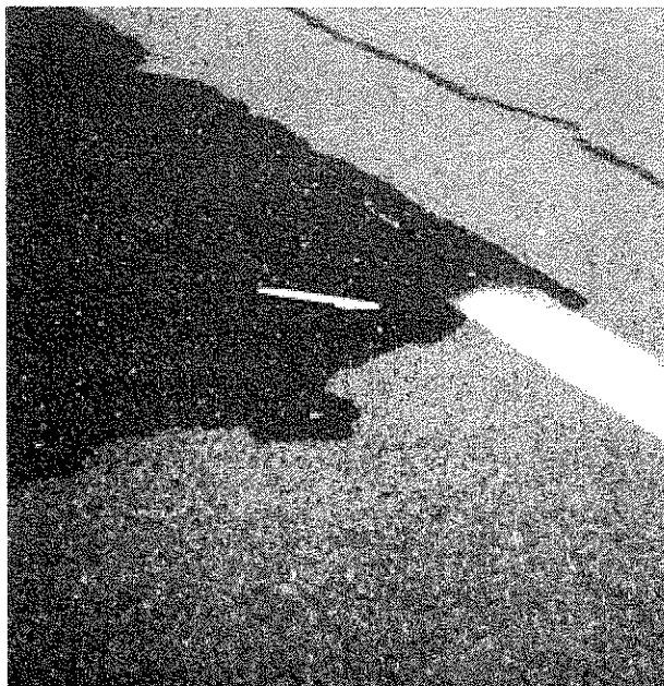
9. After rainstorm untreated pavement is still wet while pavement has dried.
