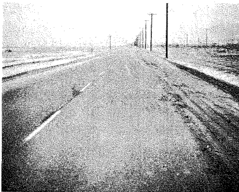
April, 1971—21 Months after Reclamite. (Approximately 1½ Hours after a Light Rain).
