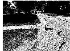
Maintenance of Traffic and resident/business access with Ogden, central sewer installation, and resurfacing will be important.
