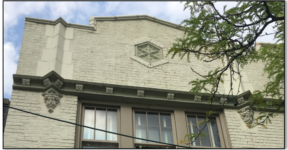
ENCOURAGED — Stone and cornice detailing.
