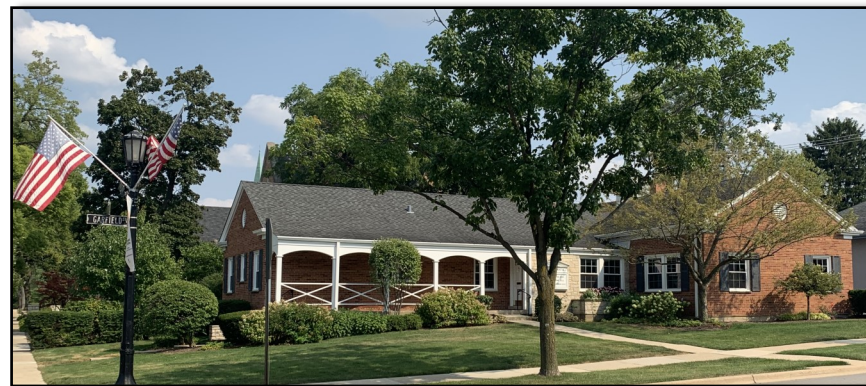
ENCOURAGED — Walkway from sidewalk to building entrance.
