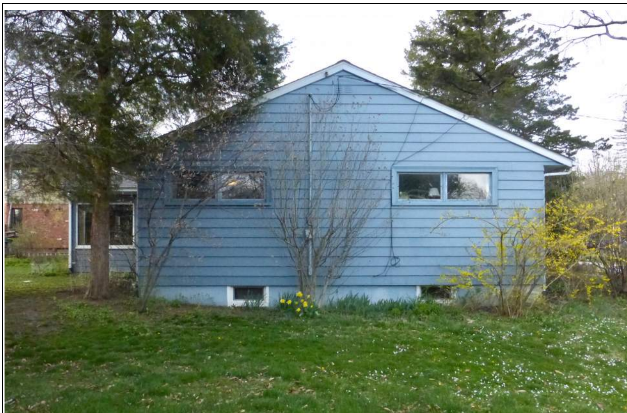
South Elevation April 14, 2020
