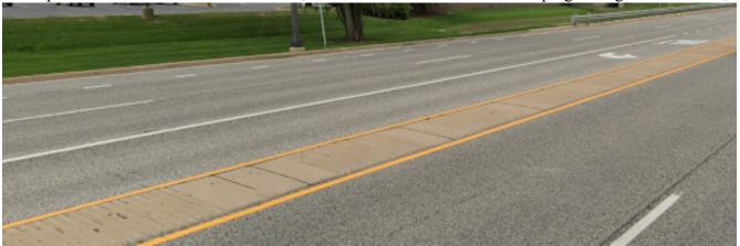
narrow mountable concrete medians would be used to define the travel lanes. These would provide the visual cue necessary to keep motorists in their proper lanes. They would also help to dissuade motorists
