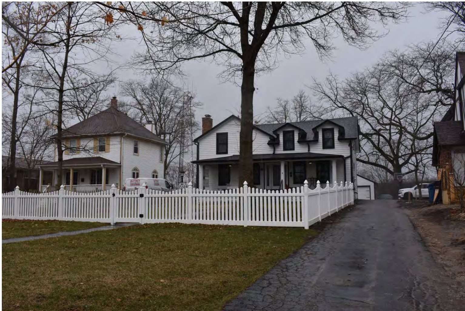
Current | View looking north from front yard of 706 Maple Avenue
