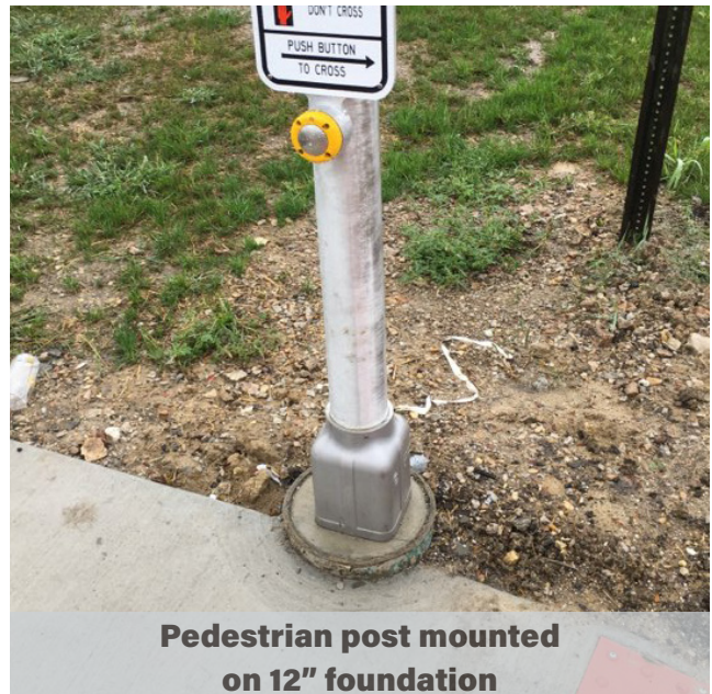
IDOT revised their standards for pedestrian post foundations from 10" to 12" to allow for mounting surface area for the pedestrian post bolt circle.
