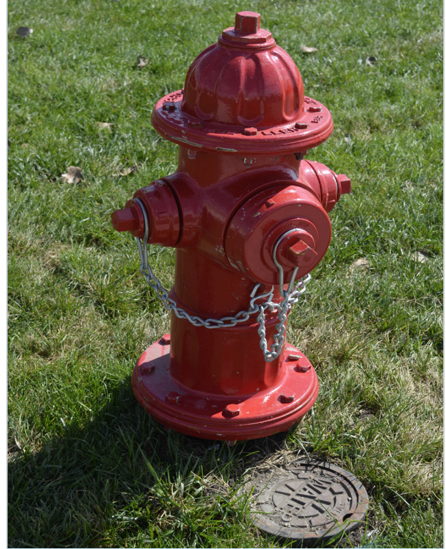
Existing utilities, such as fire hydrants, drainage structures with open grates, and other obstructions within the clear zone, must be considered.
