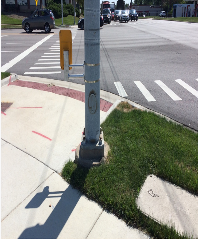
Push button extensions have been allowed to meet reach requirements, but should be avoided, if possible.
