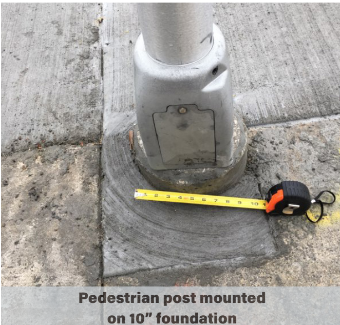
IDOT revised their standards for pedestrian post foundations from 10" to 12" to allow for mounting surface area for the pedestrian post bolt circle.
