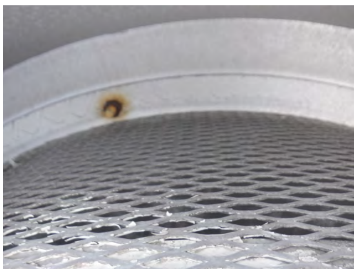
36) The vertical roof vent screen is in good condition.
