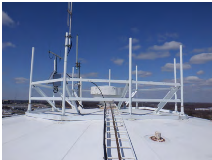
34) The roof antenna mounting structure is in fair condition.
