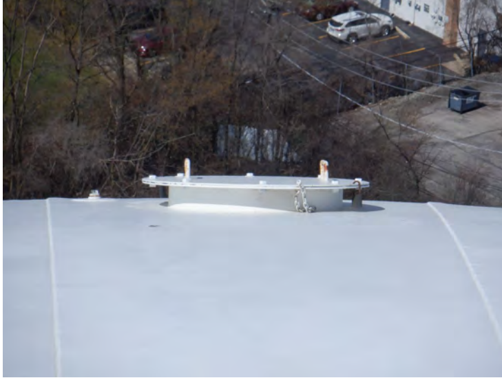
40) The bolted ventilation hatch is in good condition.
