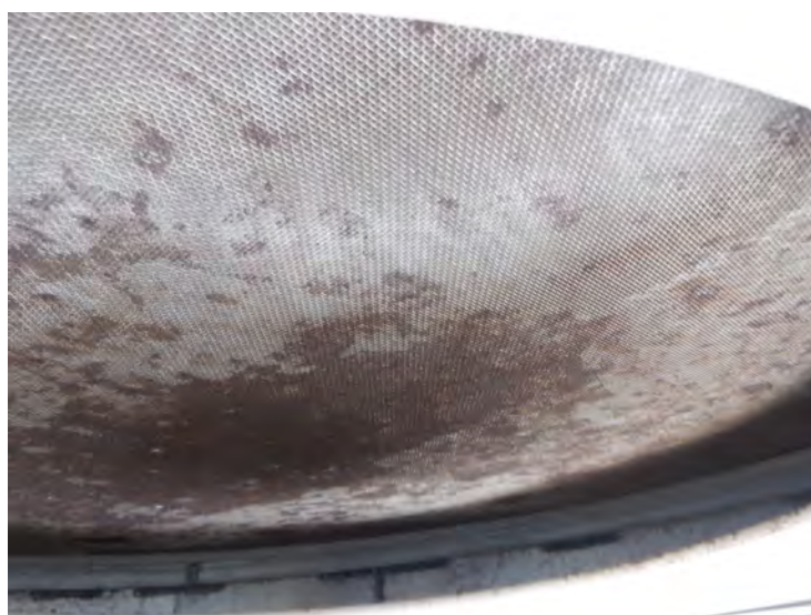
38) The inner screen in the roof vent is intact.
