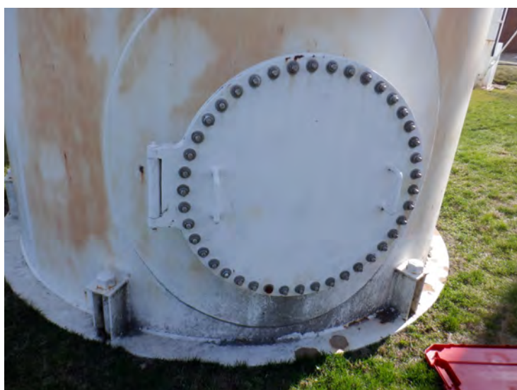
3) There are no coating failures on the riser manway.
