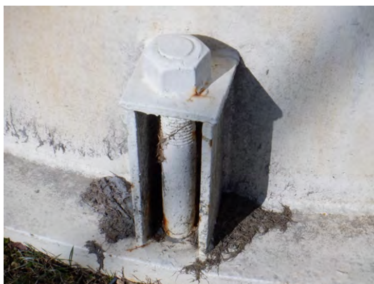
2) The riser anchor bolts are in good condition.
