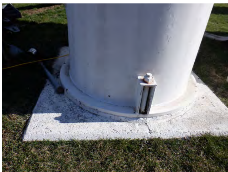
9) The leg foundations are in good condition overall. The anchor bolts are in good condition.
