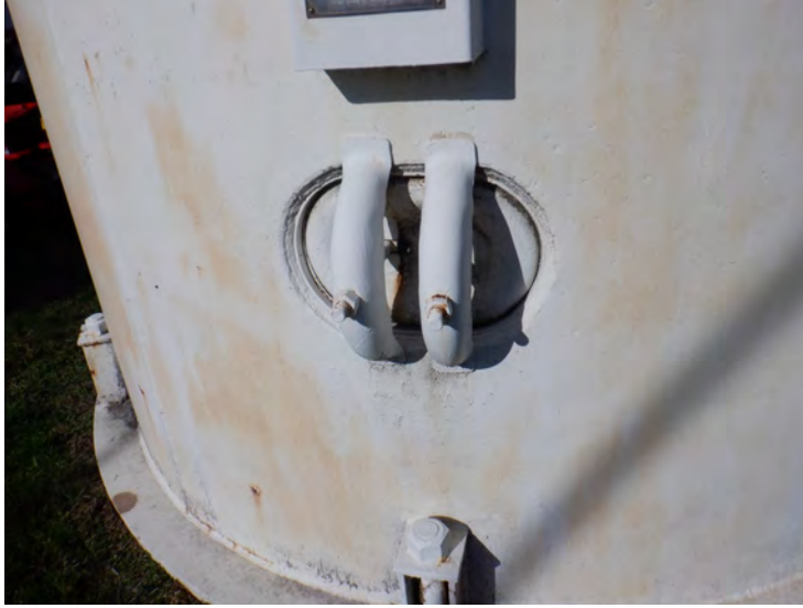
4) The secondary riser manway is in good condition.
