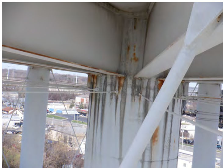
7) The riser tie rods are in good condition.
