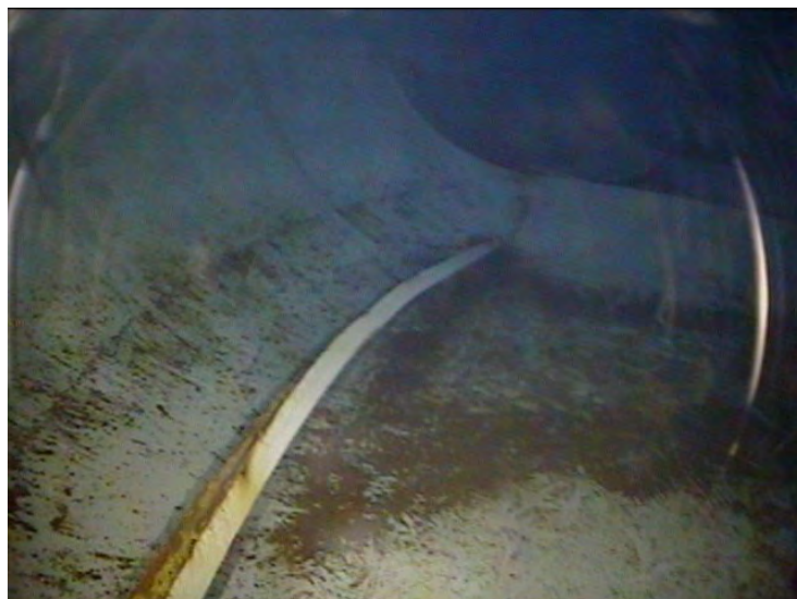
52) A piece of the sidewall stiffener/painter's railing on the floor of the tank.
