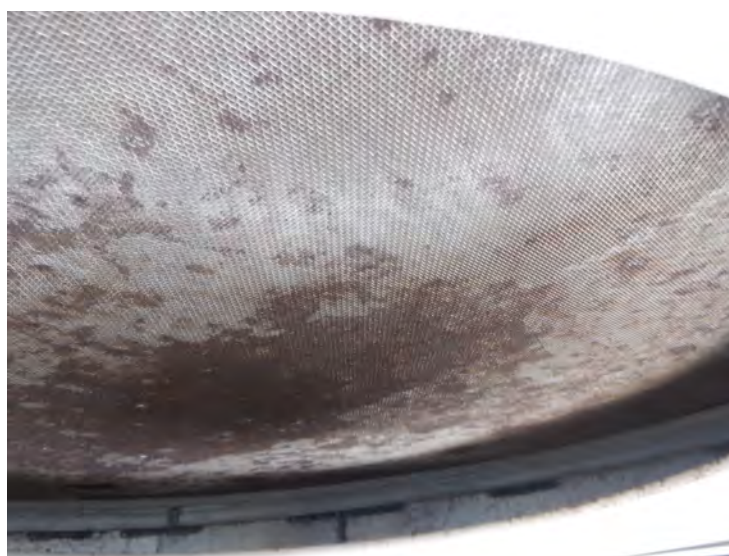
38) The inner screen in the roof vent is intact.
