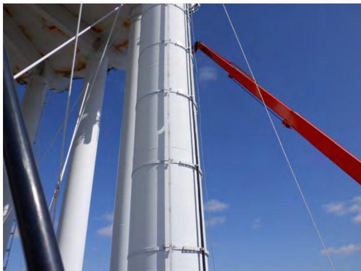
13) Band clamps attached to a leg for cable routing.
