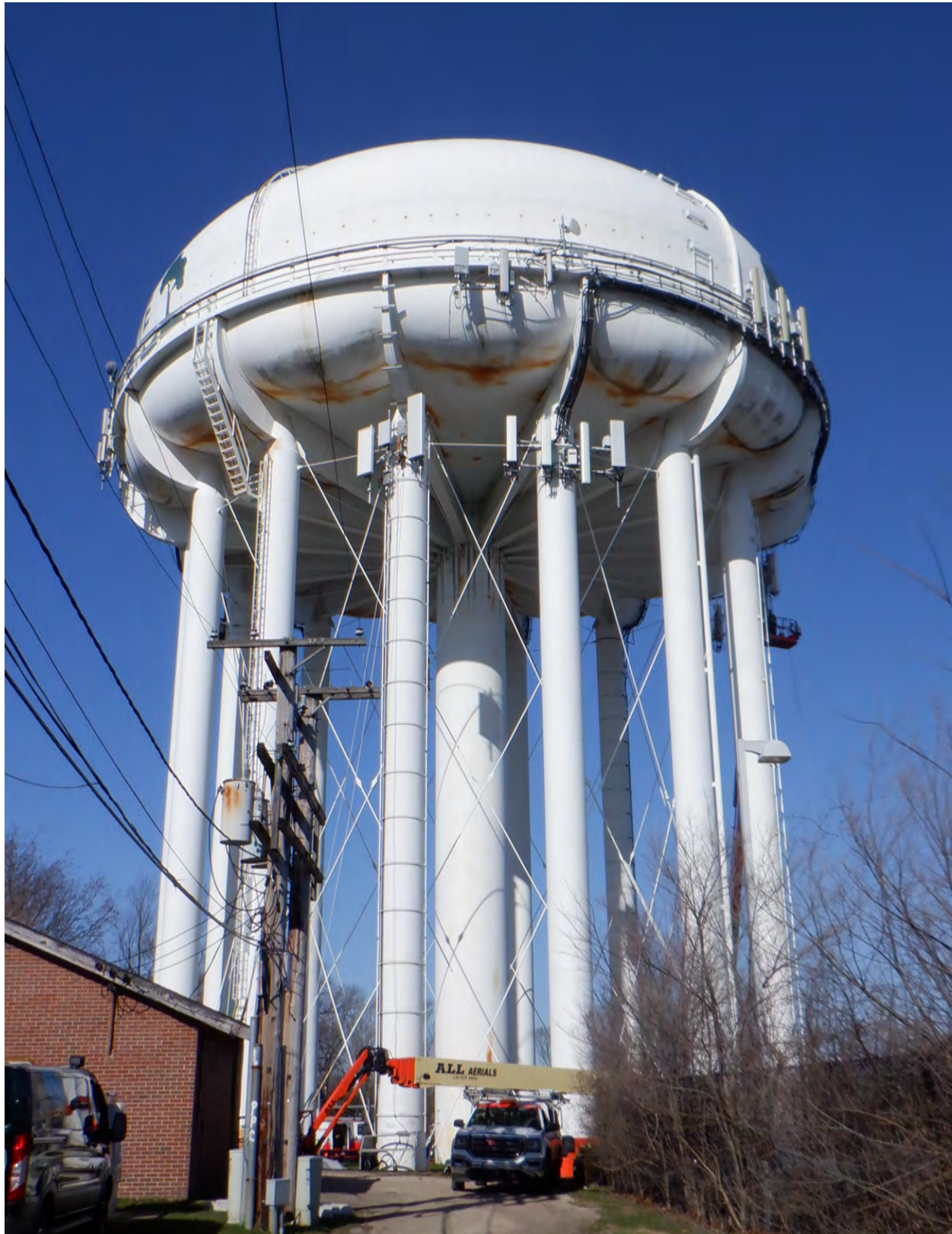
2,000,000 gallon radial arm (Downers Drive Tank) elevated water storage tank owned by the Village of Downers Grove, Illinois.
