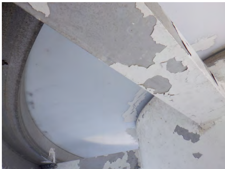
37) The roof vent pressure plate is properly aligned.
