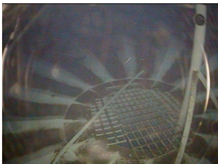
54) There is a grate over the riser in the wet interior.
