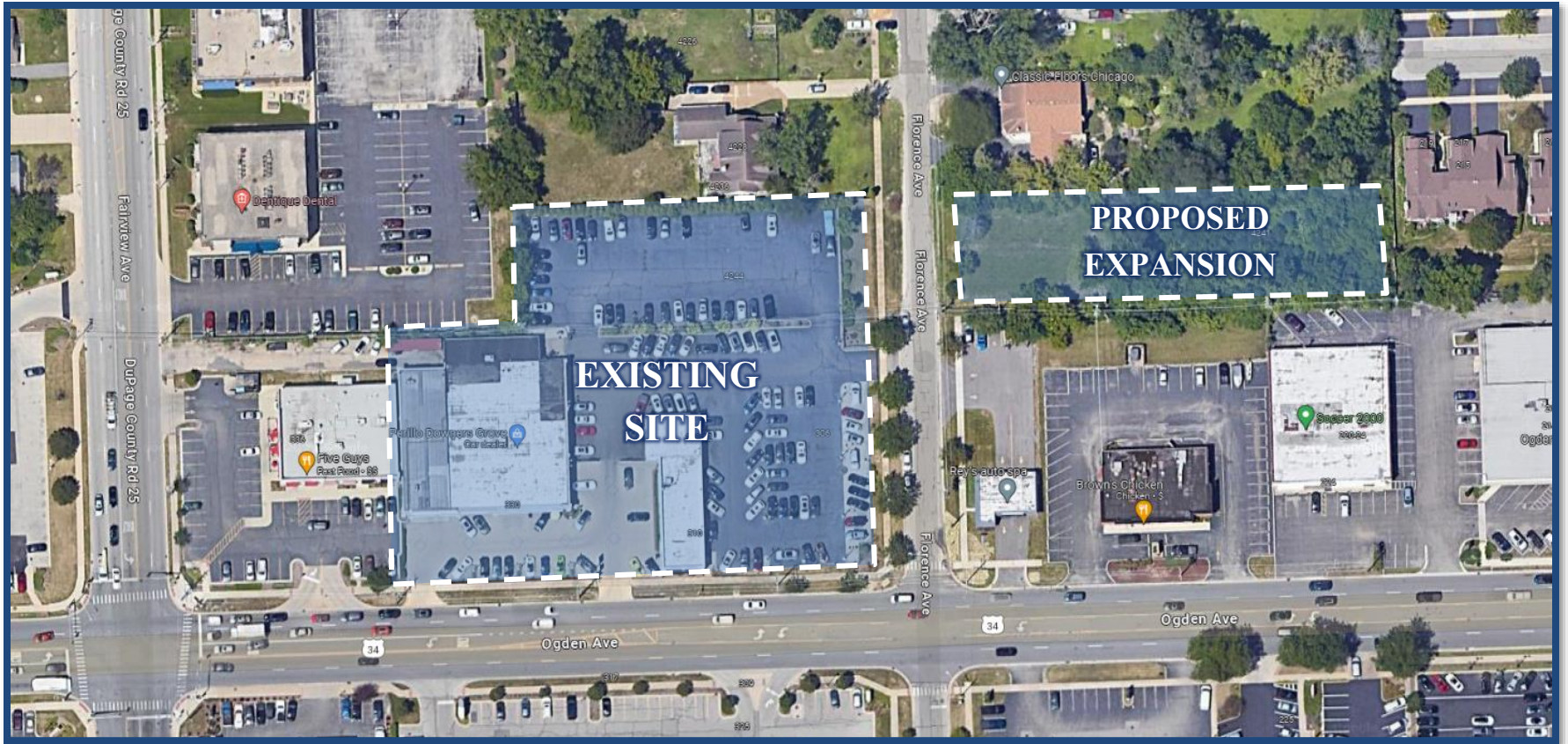
Aerial View of Site
