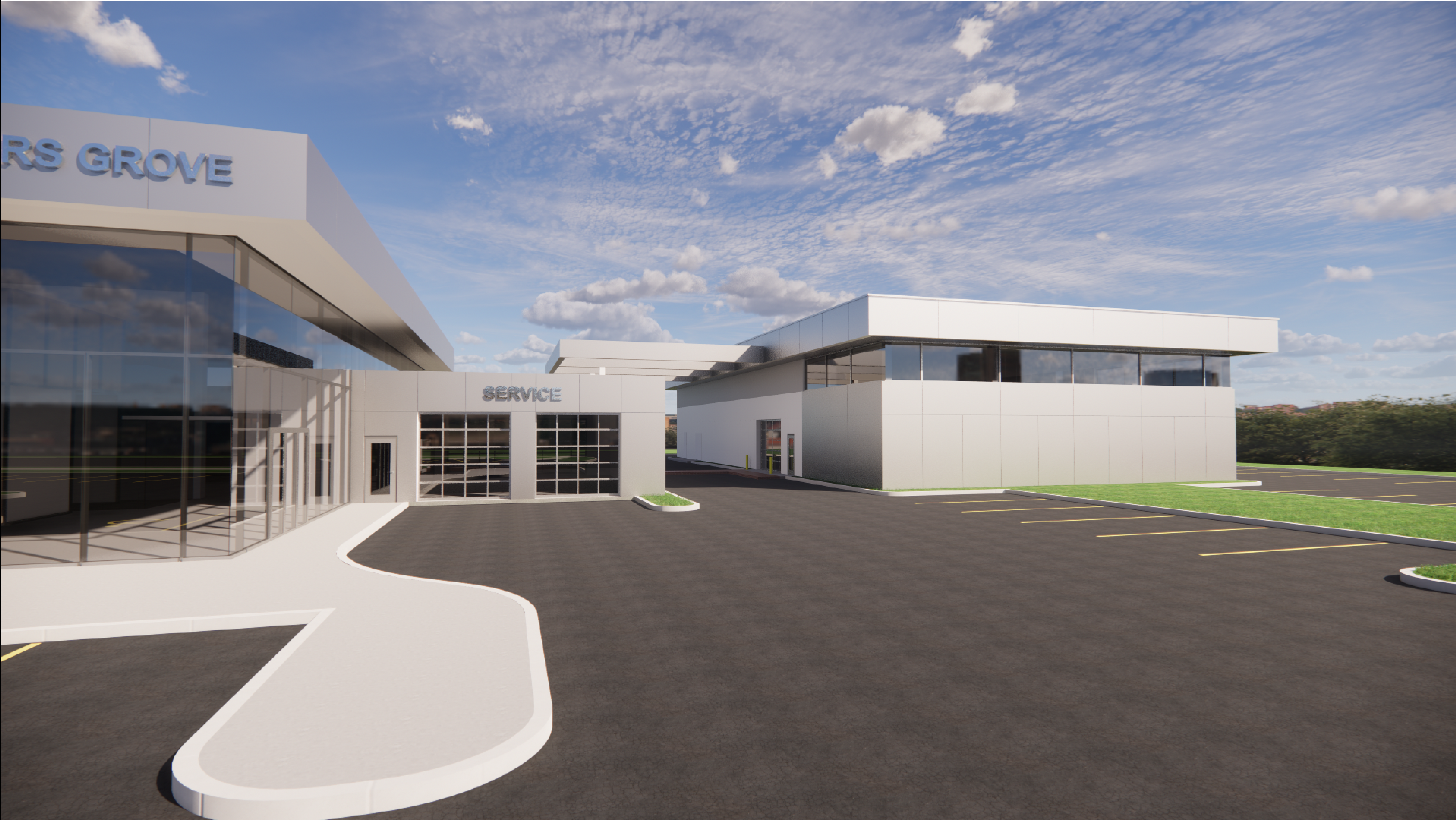
VIEW 004 - LOOKING NORTH FROM OGDEN AVE
