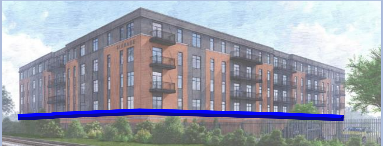
North and West Facades
