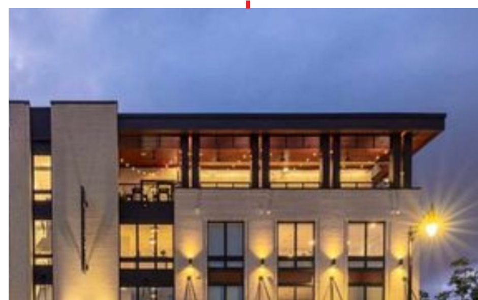
FORMED METAL ROOF OVERHANG CREATES DISTINCTIVE CAP TO BUILDING WHILE SHADING TERRACES FROM AFTERNOON SUN
