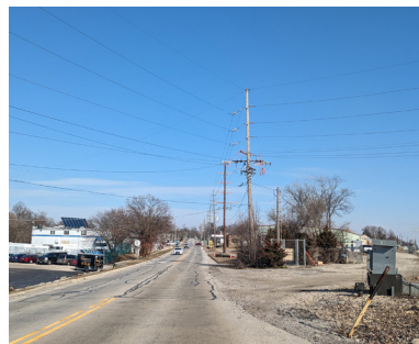
Rail crossing conditions at Maple Avenue
