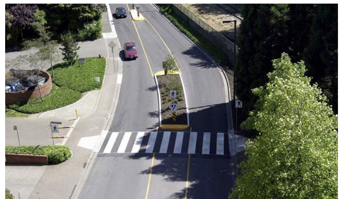
An example of a piano key crosswalk Source: CMAP
