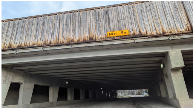
Underpass conditions at Jackson Drive and I-355 leading into Downers Grove. There is minimal lighting and pavement is damaged due to run-off
