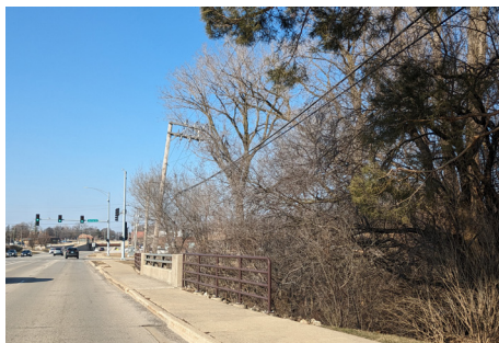
Bridge along Belmont Avenue
