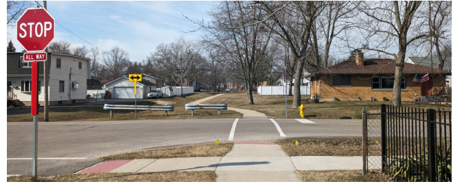
New ADA compliant crossings
