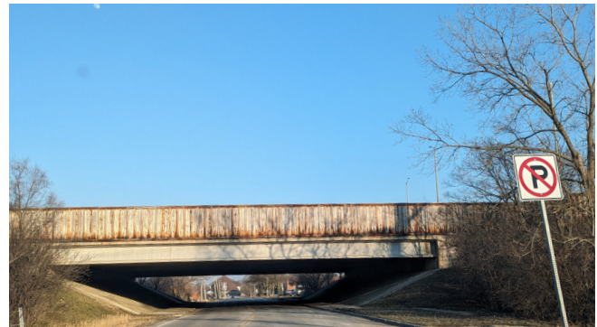
Underpass conditions at Hitchcock Avenue and I-355. There are no continuous sidewalks or bridge lighting. Utilities are adjacent to the road edge and debris was observed along the pavement edge.
