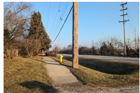
Debris and buckling on Warren Avenue
