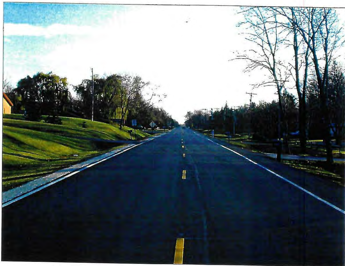
(Clarendon Hills Road looking south)
