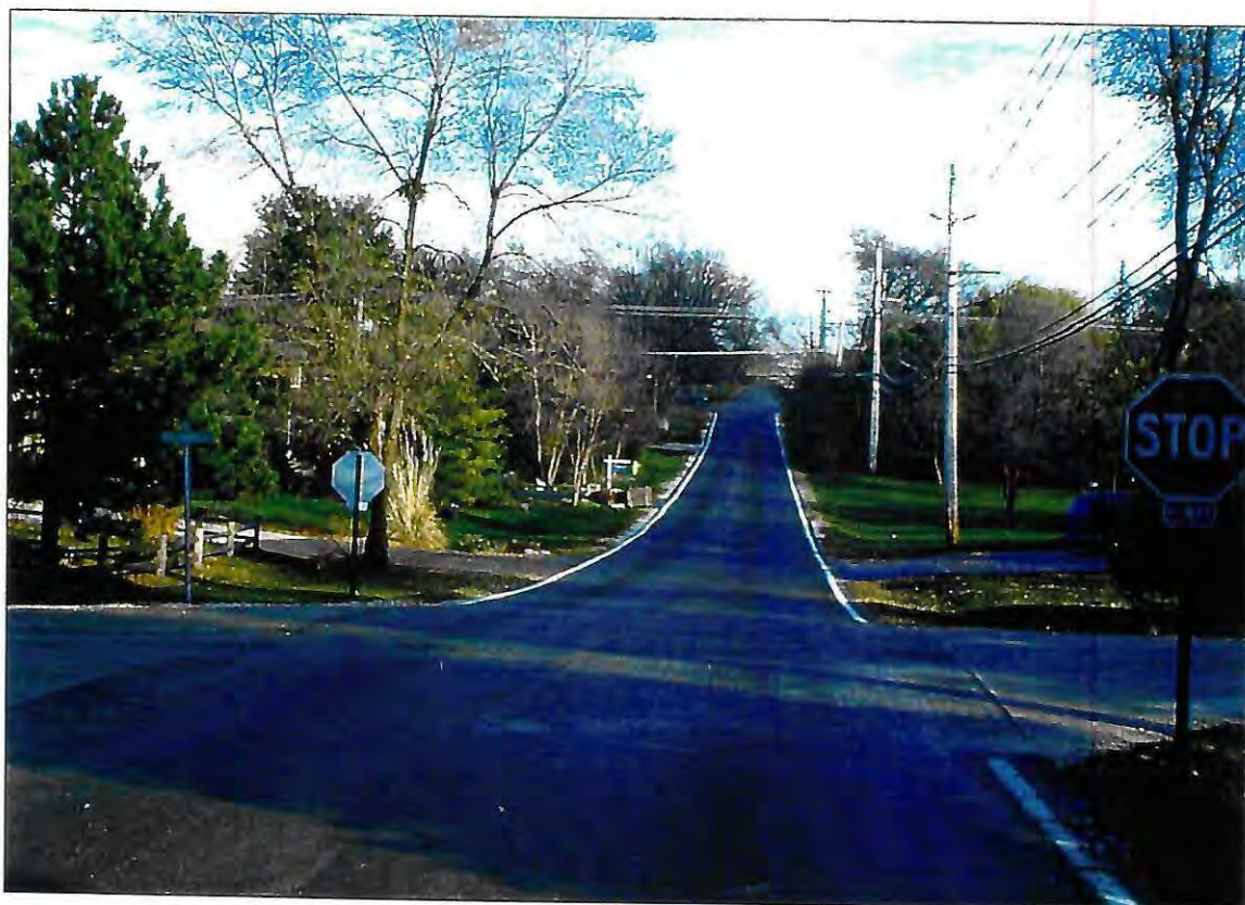
(59 th Street looking east, just east of Belmont Road)
