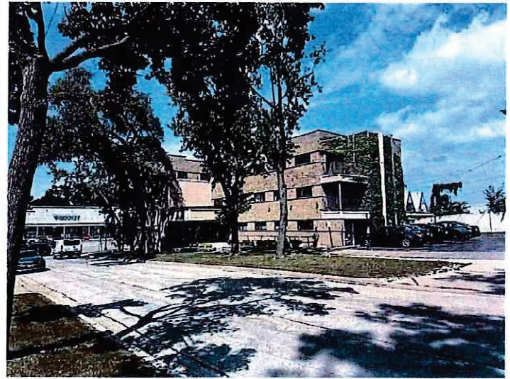
View to Northeast
