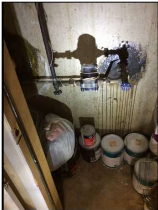
Pre Installation Photo
