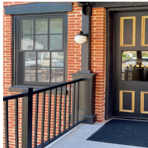
BLACK METAL RAILINGS
