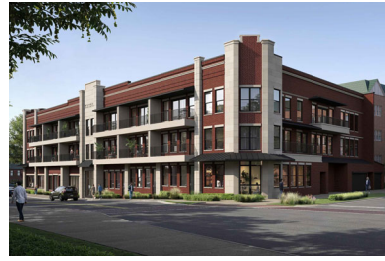
NORTHEAST CORNER LOOKING SOUTH
