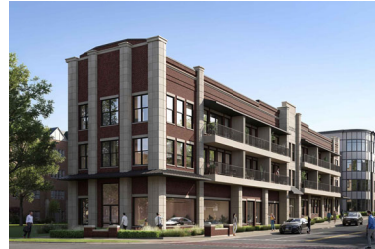
SOUTHEAST CORNER LOOKING NORTH
