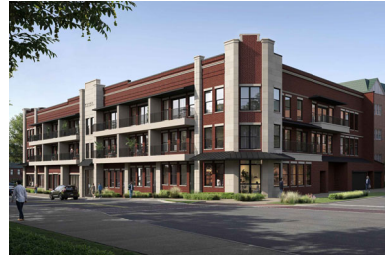
NORTHEAST CORNER LOOKING SOUTH
