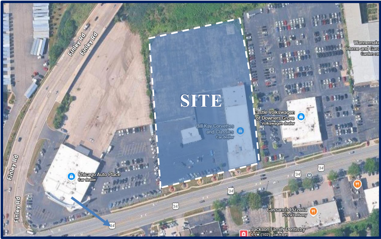
Aerial View of Site
