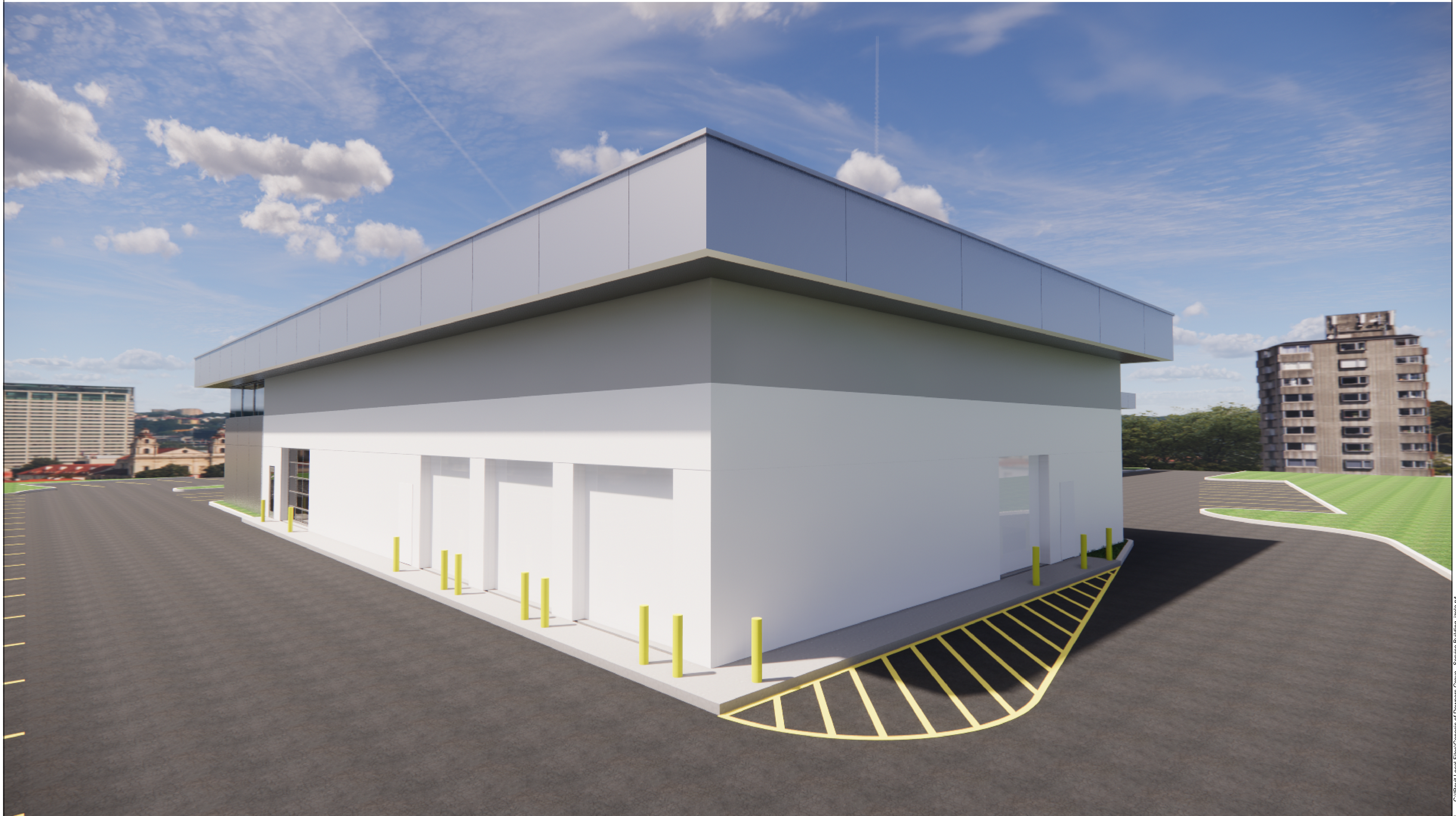
VIEW 005 - LOOKING SOUTH TOWARDS NE CORNER OF PROPOSED SERVICE BUILDING
