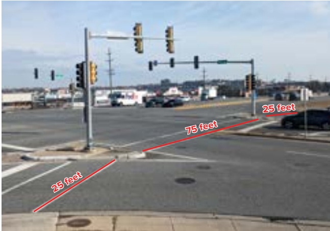
Finley Road at Butterfield Road facing northeast
