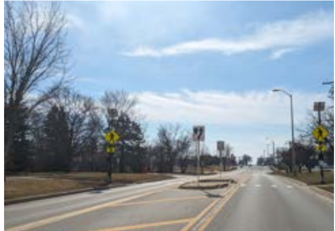
Existing Fairview Avenue mid-block crossing near Westwood Park
