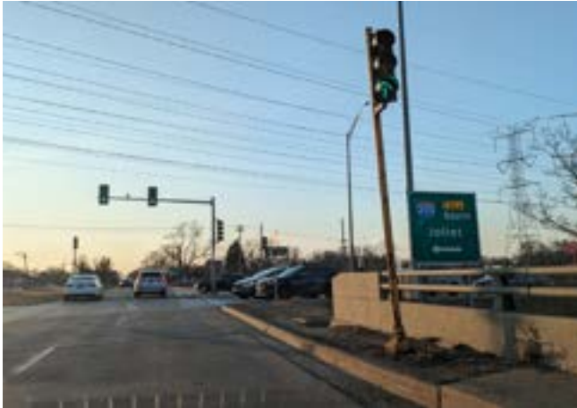
Bridge crossing conditions at Maple Avenue and I-355
