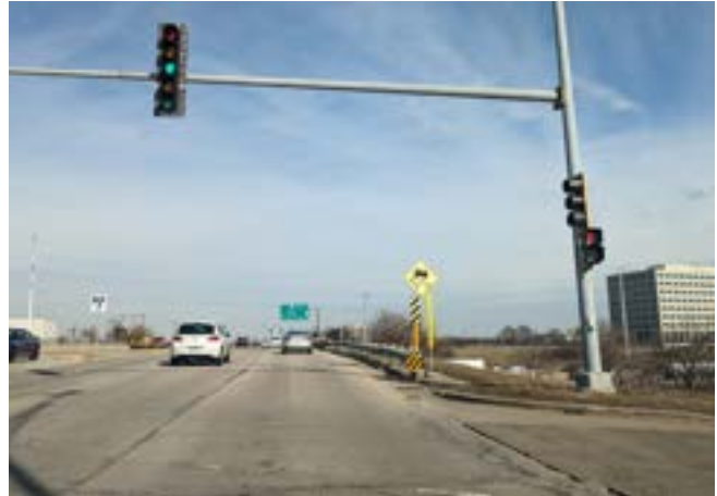
Bridge crossing conditions at Warrenville Road and I-355
