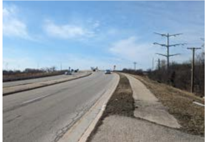
Narrow Finley Road sidewalk and bridge, facing south towards I-355
