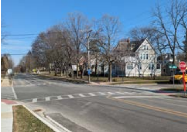
Example of newly painted piano key with double-bar crosswalks at Maple Avenue and Washington Street
